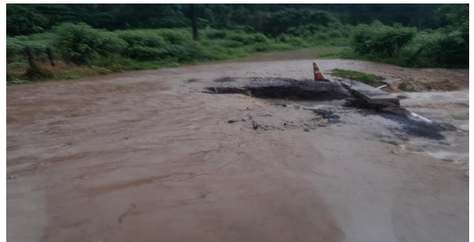
Figure F: Namaqumaqua Crossing, Navua on the 22 nd . Source: Fiji Roads Authority.
