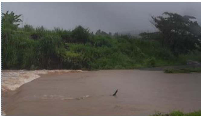
Figure G: Wainibuka crossing, Colata Cocoa Road on the 25 th . Source: Fiji Roads Authority.
