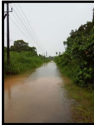
Figure 1 Flood prone road in Aimeliek from May 1st rainfall
