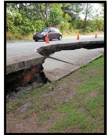
Figure 2 Damage to cracked road in Airai from rainfall on May 1 st .
