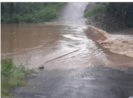
Figure 18: Navula Road in Ba inundated with floodwaters on 13 th December, 2022. Source: Fiji Roads Authority
