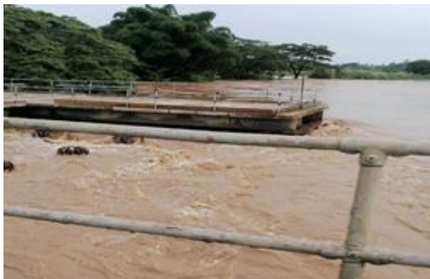
Figure 22: Rising flood waters at the Navo Bridge in Nadi on 31 st December, 2022. Source: fijivillage
