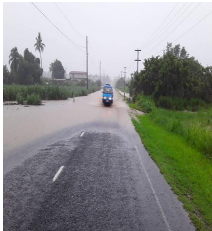
Figure 16: Kings Road in Rakiraki inundated with floodwaters on 13 th December, 2022. Source: Fiji Roads Authority
