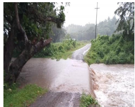
Figure 20: Lawai Crossing in Sigatoka inundated with floodwaters on 30 th December, 2022. Source: Fiji Roads Authority
