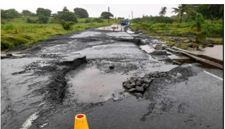
Figure 7: Rabulu road (Tavua) damaged due to continuous flooding on 17 th February, 2023. Source: fijivillage.
