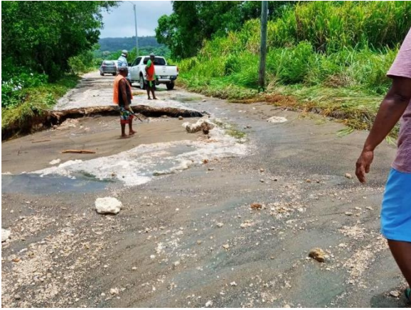
Damage to Roads, Devil's Point, Port Vila Date: 5 th February 2021,
