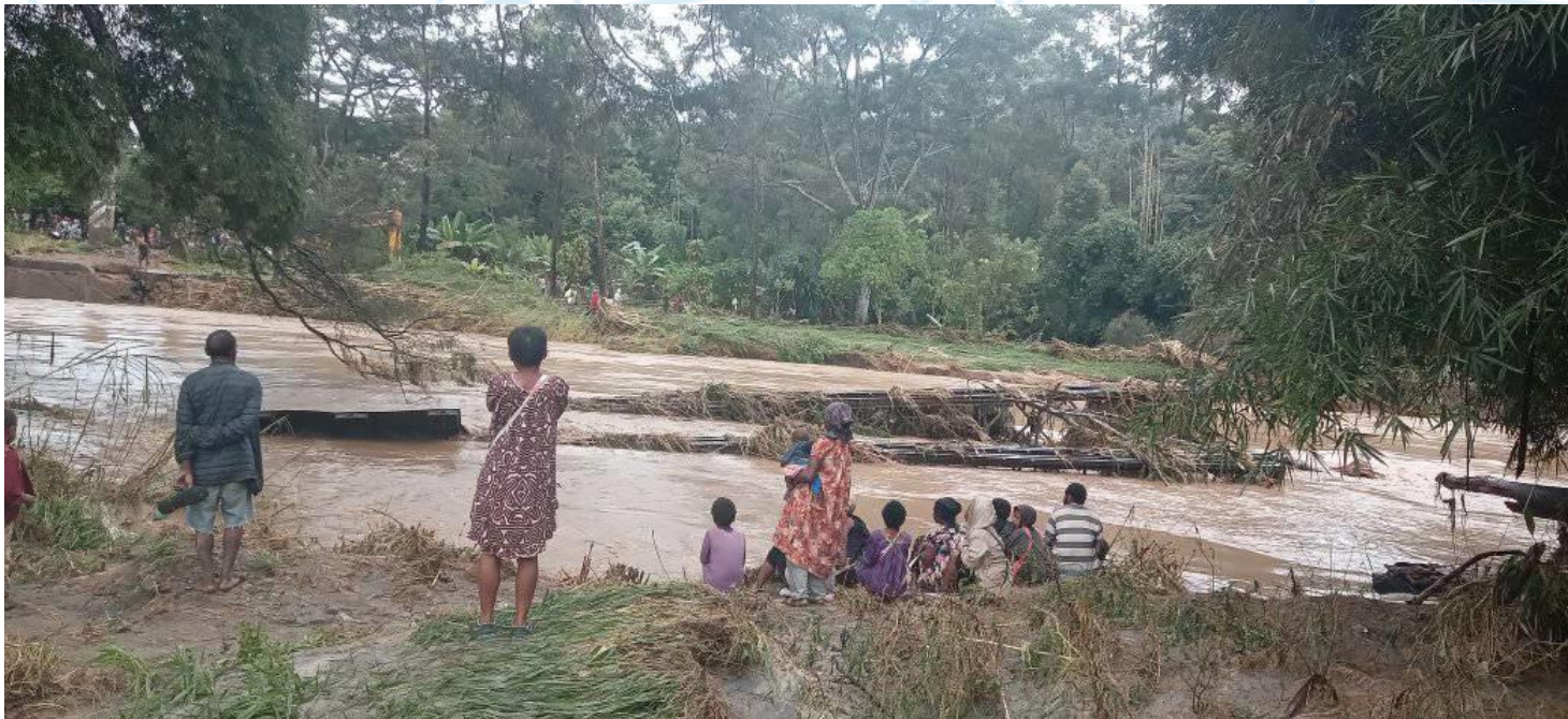
Helpless onlookers watch as Marasin Bridge swept away by floods
