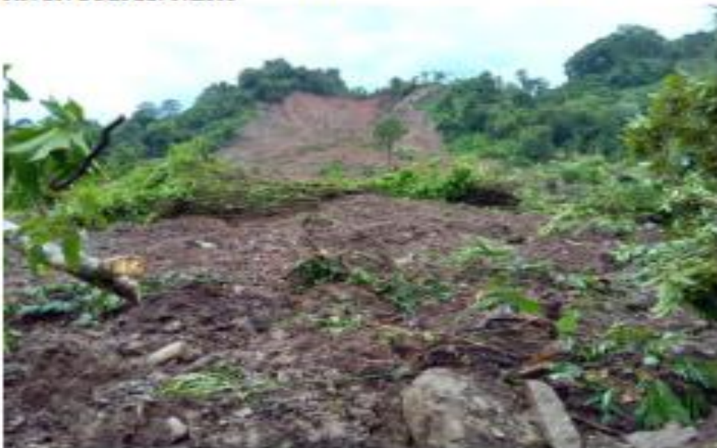
Landslide at Kuratidalo Village, Small Ngella causing damage to a dwelling house and kitchen. Source: P-DOC CIP
