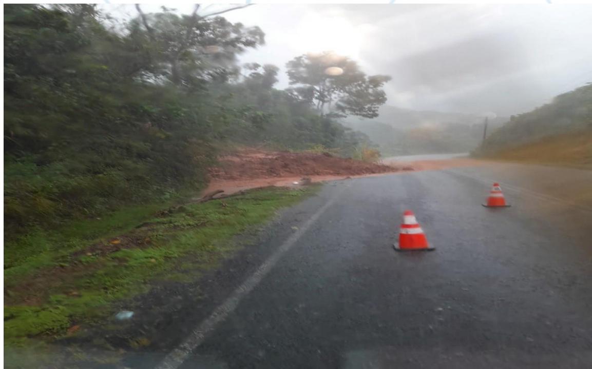
Landslide along Queens after Nakorovou in Central Division on 18th December, 2023. Source: Fiji Roads Authority
