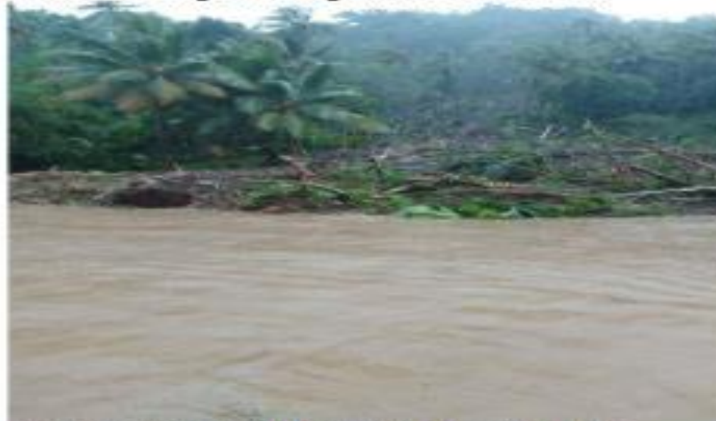
Landslide at Sagana Village. Source: Fredrick Dotho
