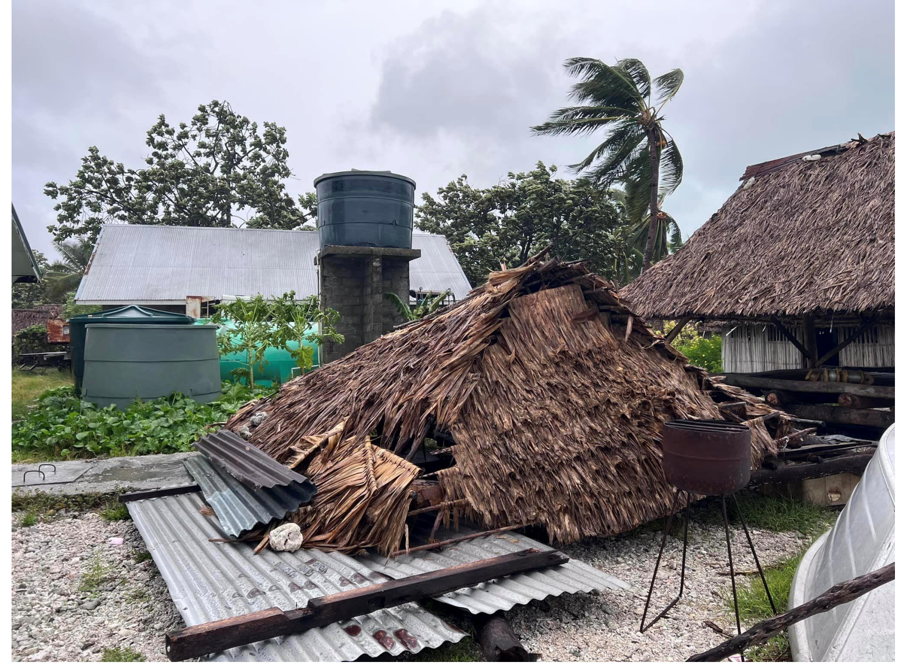
Right: Local house destroyed by the strong wind on Marakei island.
