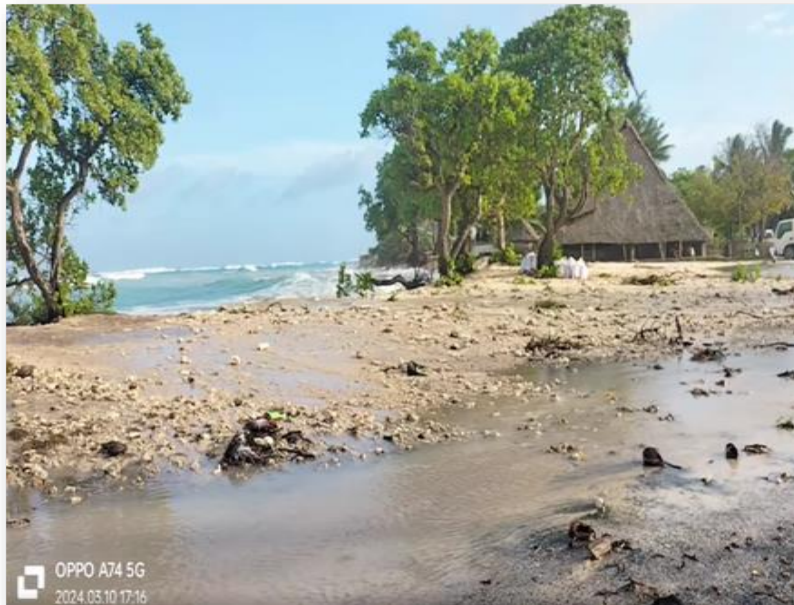
Top images: Left. Coastal overtopping to the public road and gathering place (Maneaba) at Temaiku. Right. Central island, Abemama coastal flooding at the church compound.
