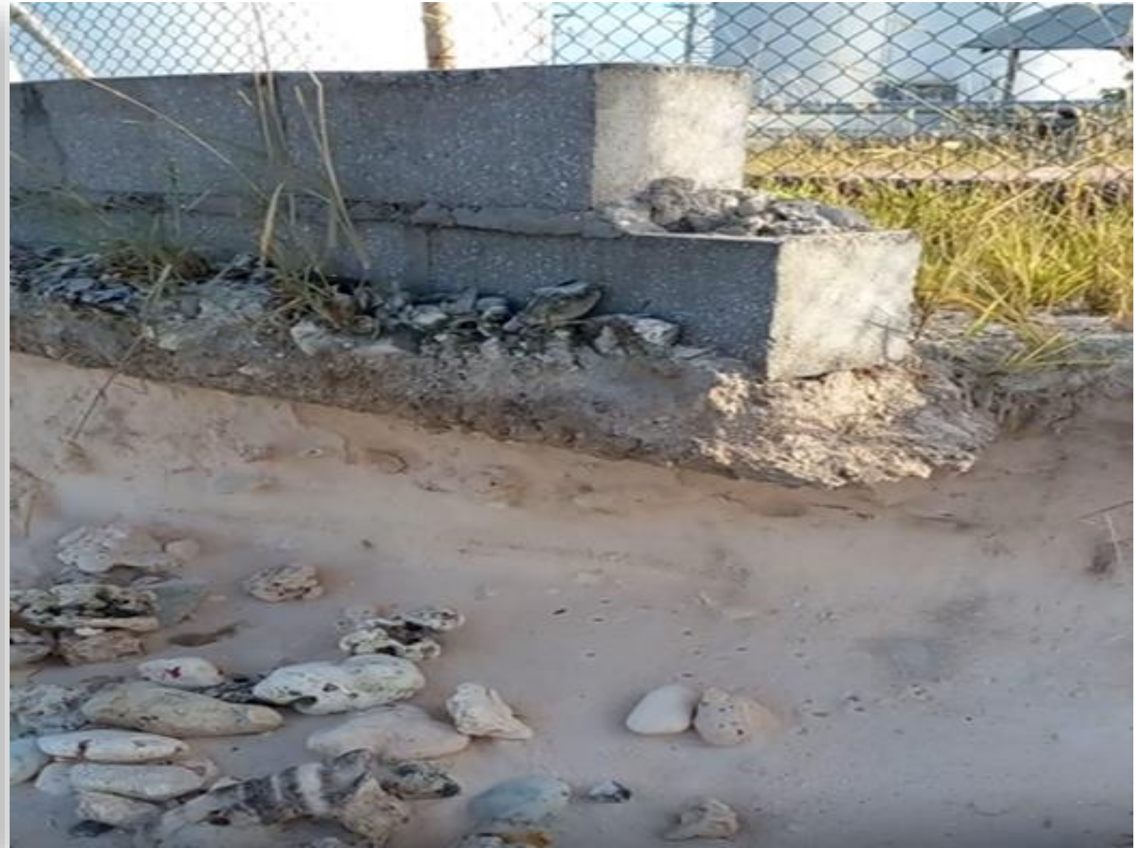
Left and Right images: Destruction to the Kiribati Oil Company Limited (KOIL) seawall at Kiritimati in the Line Islands.
