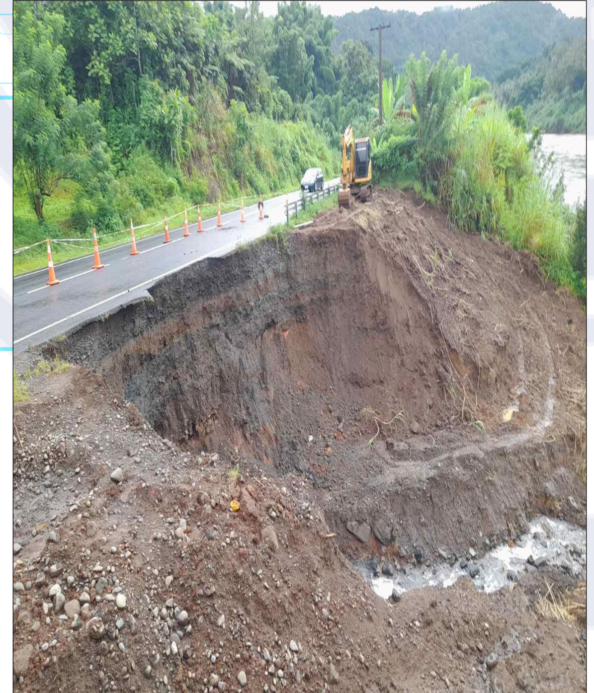
A road dropout occurred in Nabulini in the Central Division on 25 th December during a period of heavy rainfall.
