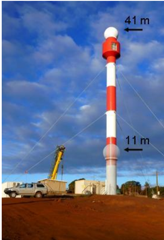
Raising the elevation of Tiebaghi meteorological radar (from 11 m to 41 m at the top)
