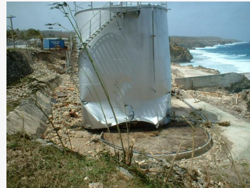
Tank moved by extreme wave, TC Heta (Source: Niue Met Service)
