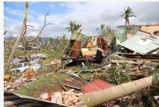
Wind damage from TC Winston, Fiji (source: ABC News Australia)
