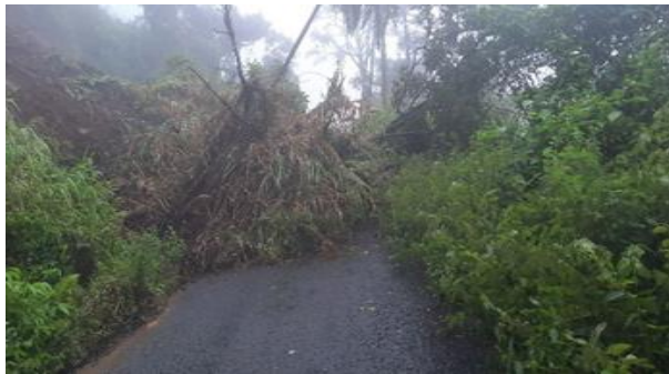
Landslide in Nadarivatu (Western Div.) - 18 th Feb 2023 (Source: Fiji Roads Authority)
