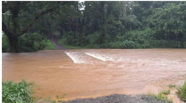
Qelemumu Crossing in Wainikoro (Northern Div.) – 11 th Jan 2023 (Source: Fiji Roads Authority)
