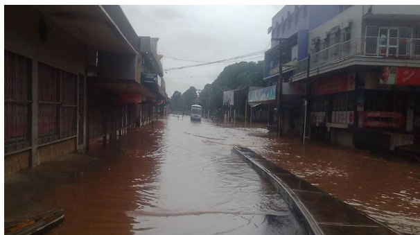
Flooding in Nadi town (Western Div.) – 6 th Mar 2023 (Source: fijivillage)
