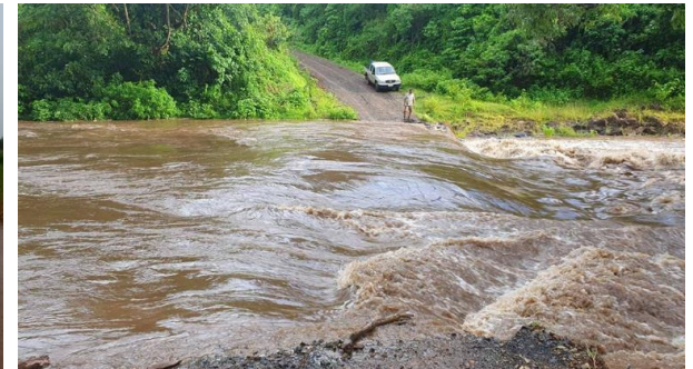
Flooded Banikea Crossing on Kavula Road, Lekutu, Bua (Northern Div.) – 28 th Jan 2023 (Source: Fiji Roads Authority)
