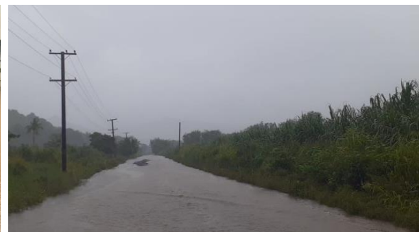
Flooded Waimari Road in Rakiraki (Western Div.) – 7 th Mar 2023 (Source: Fiji Roads Authority)
