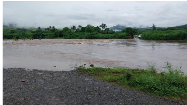
Toge Crossing in Ba (Western Div.) – 5 th Jan 2023 (Source: Fiji Roads Authority)
