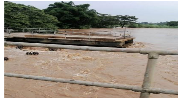
Rising flood waters at Navo Bridge in Nadi (Western Div.) – 31 st Dec 2022 (Source: fjjvillage)
